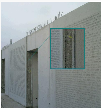
Insight in a prefabricated wall
