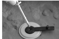
Remove rod after concrete hardens
